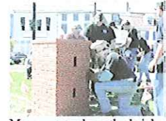
Mason at work on the brick pillar
